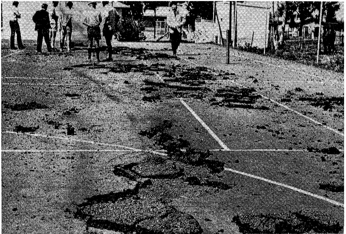
"Sucked Up" surface of tennis court showing extensive damage— at Rosemead, South Africa.
