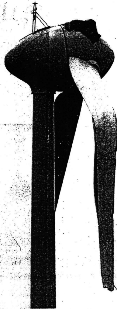
The wrecked wind turbine - minus one rotor - in Conisholme. Metal fatigue and ice are now the main suspects, rather than a UFO Photograph: Chris Radburn/PA
